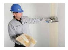
Two or three further applications of jointing compound are trowel applied, each feathered out beyond the previous application. An equal number of applications are made to spot screw heads. Once dried, the joint treatment is sanded as necessary to achieve a smooth surface.
