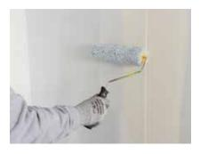
Gyproc Drywall Primer or Gyproc Drywall Sealer is applied to the entire board surface and jointed areas, to prepare the lining for final decorative treatment.
