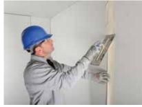
For external corners Gyproc Corner Tapes are bedded with a Gyproc setting compound.
