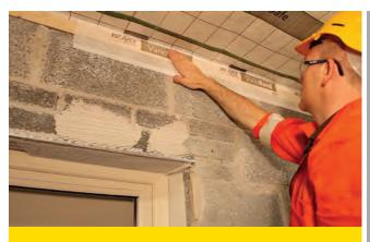
Timber wall plate to block junction
