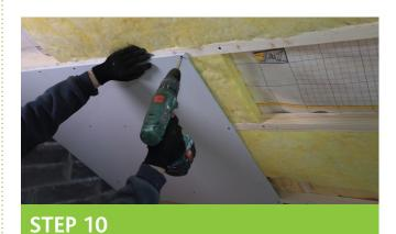
Finally use Gyproc Plasterboard applied to counter battens to complete the installation.
