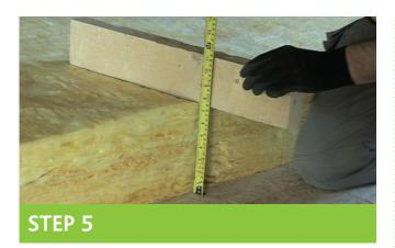
Unroll it to allow full thickness recovery and then cut to length using a straight edge to help ensure a clean straight cut.
