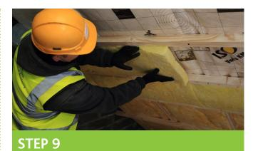
To increase U-value performance friction fit additional 50mm Metac between the counter battens.
