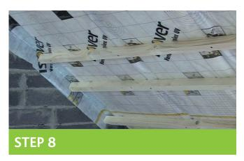
ISOVER recommends best practice by installing 50x50mm counter battens in the opposite direction below the rafters. This creates a service zone without the need to penetrate the Vario membrane.
