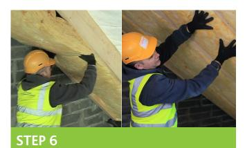
Push and friction fit the insulation in between the rafters (taking care not to compress it) keeping Metac flush with the face of the rafters.
