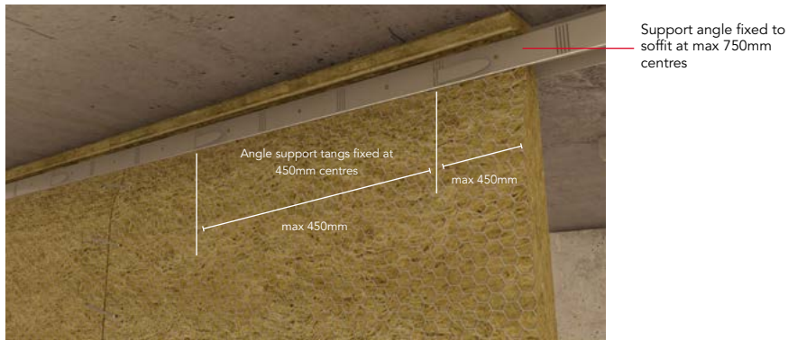
Figure 10 50mm Fire Barrier fixed to concrete soffit.
