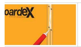
Prior to installing any cladding material (siding, metal, wooden, decorative brick veneer, etc...) on **BoardeX** surface, an appropriate sealant should be used in the joints of **BoardeX**, in order to prevent air, moisture and water from leaking into the system.
